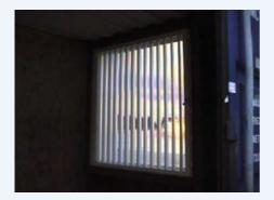
The way the Blast protection blinds protect is deceptively simple. The second a blast occurs in the vicinity of your protected premises, the blades snap shut. This provides an impenetrable barrier, preventing flying glass and debris from penetrating the building, protecting both the internal premises and individuals in them. The building also remains secure from looting.
